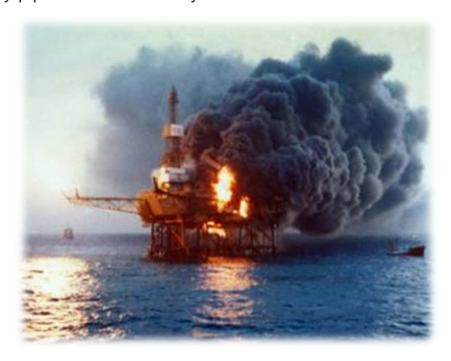
The original modules on the structure were carefully located, with the staff quarters kept well away from the most dangerous production parts of the platform. But this safety feature was diluted when the gas compression units were installed next to the central control room. Further dangers arose when Occidental decided to keep the platform producing oil and gas as it set about a series of construction, maintenance and upgrade works.
